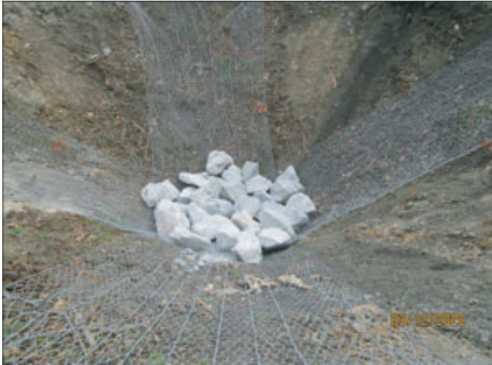
Ring netting and riprap
