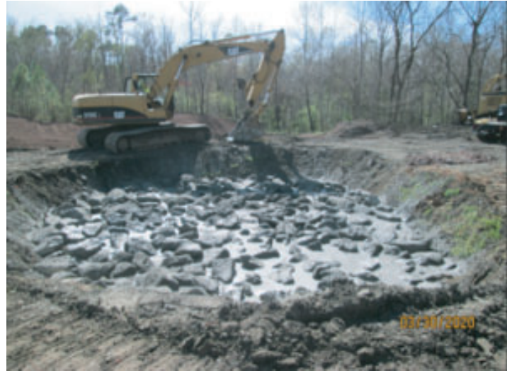
Top layer of riprap & grout
